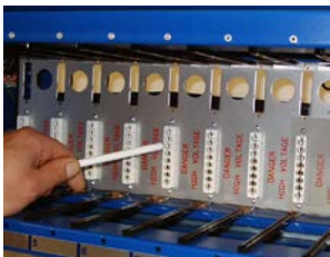
Step 1: Verify installation of contact.
